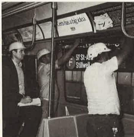
Supervisor Mike Casaula makes notation on checklist as Car Inspectors Varghese Daniel (left) and Sivaraman Nair (right) change the side sign.
