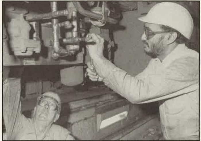
At the Jerome Shop, Car Inspectors Frank Doolan (under car) and Narayanankutty Karat tighten the last bolts on the newly installed air brake valves.
